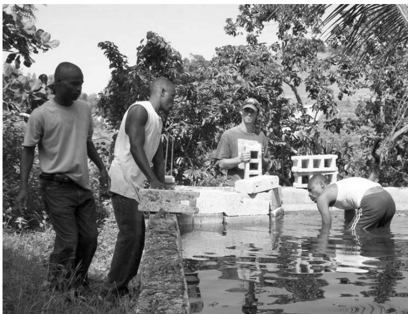
Nick Warren helps Haitian villagers build a fish pond.
